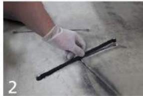
2 Press the CCL into the epoxy
