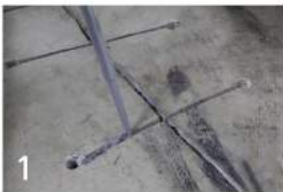
1 Fill cut with DUNLOP BUILDER'S BOND
