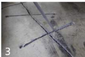
3 Apply additional epoxy over the CCL
