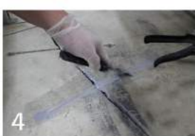
4 Scrape away excess epoxy and smooth surface
