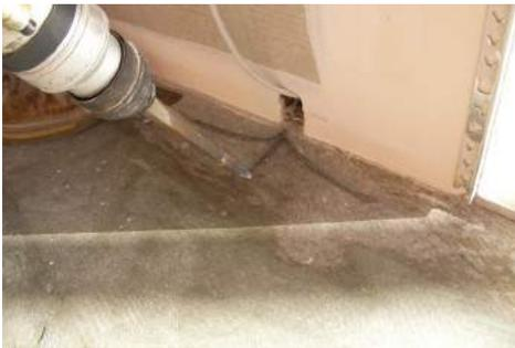
*Marking out the cold tail channels*
