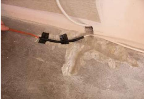
Then start spreading the element around the floor using the jig you cut earlier.
